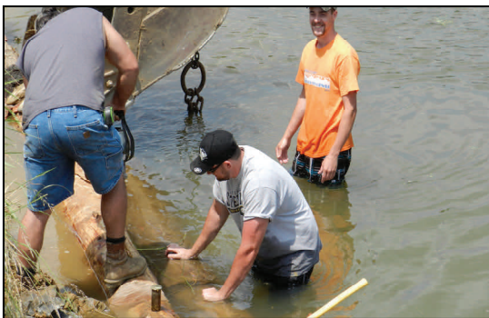
In Progress: log deflectors being placed in stream.
