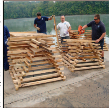
Volunteers construct porcupine cribs at Hinckston Run Dam
