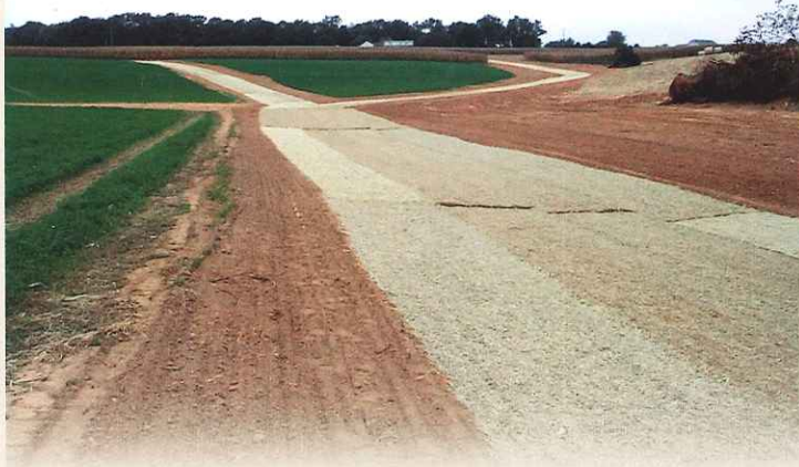
Newly constructed grass waterway
