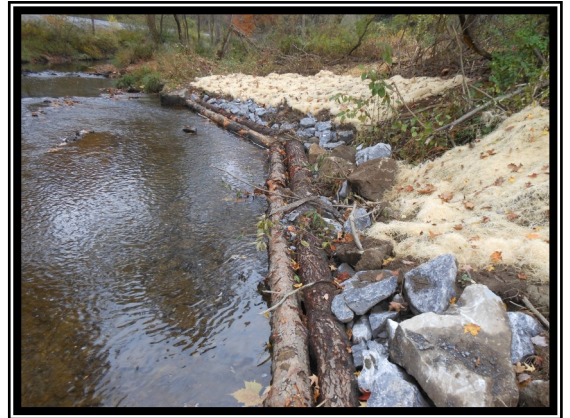
Modified mud sill installed to provide streambank stabilization and overhead cover for fish. The erosion control blanket helps to keep seed in place until growth begins.
