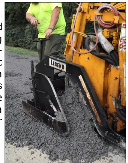
Seen at right, township officials laying Driving Surface Aggregate with a paver.
