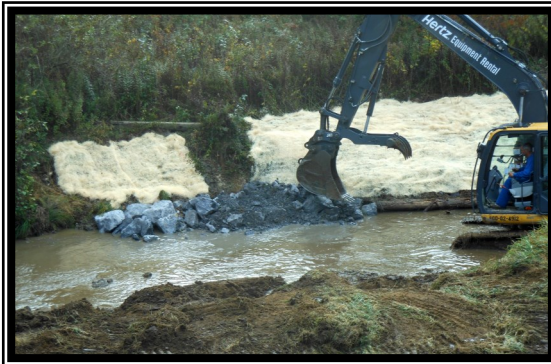
Construction of a mud sill.
