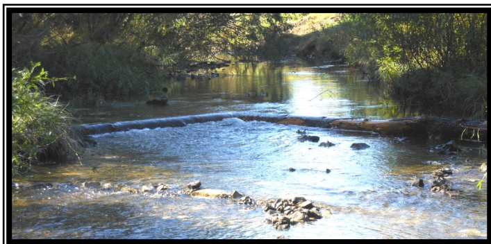
Log Cross Vane takes water to the center of the channel to raise the oxygen levels for aquatic life.
