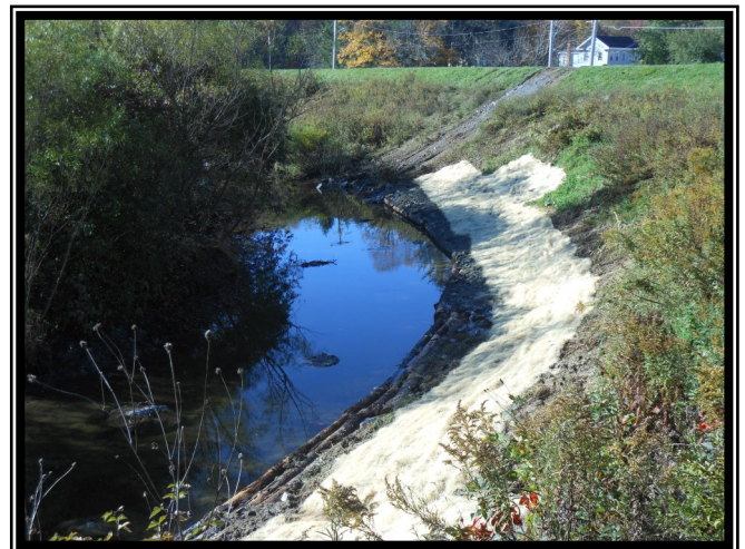
Last mud sill completed before the railroad bridge in Cherry Tree.
