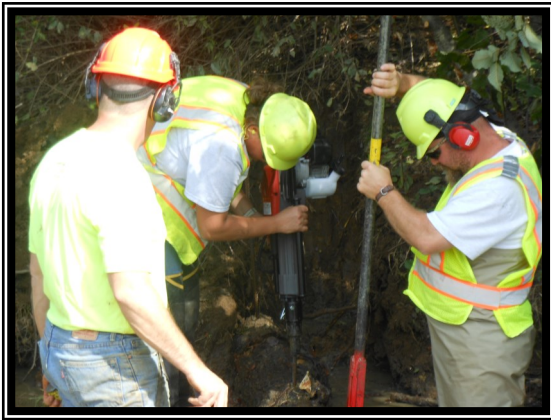
Installing rebar for log placement
